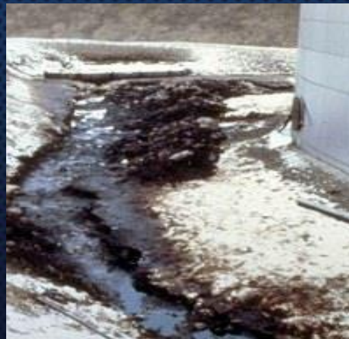
LEAKAGE LEADING TO ENVIRONMENTAL POLLUTION
